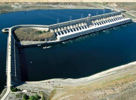
Chief Joseph Dam spans the Columbia in northwest Washington
